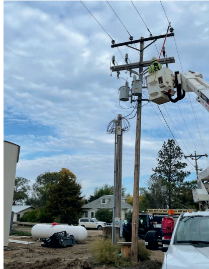
Line crew installing a new service in Reliance.
