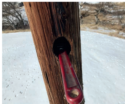
Pole scheduled for replacement due to woodpecker damage.
