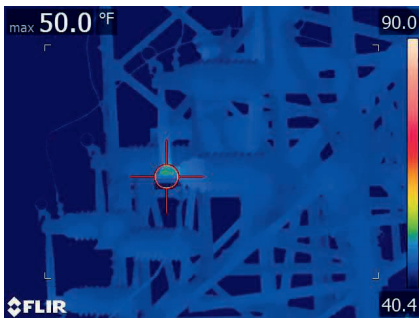
Infrared thermal imaging in the winter months can show potential problems by finding loose connections.
