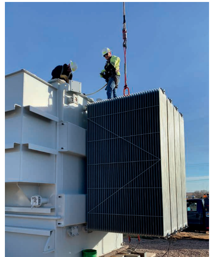
Murdo crew prepping the Keystone XL substation transformers to be hauled away.
