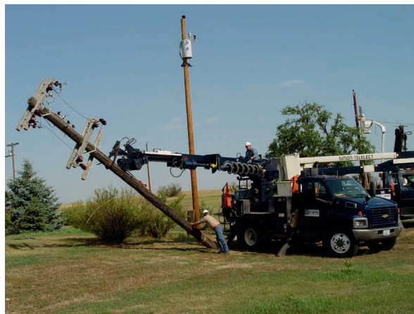
Lyle operating the digger truck on a pole change.
